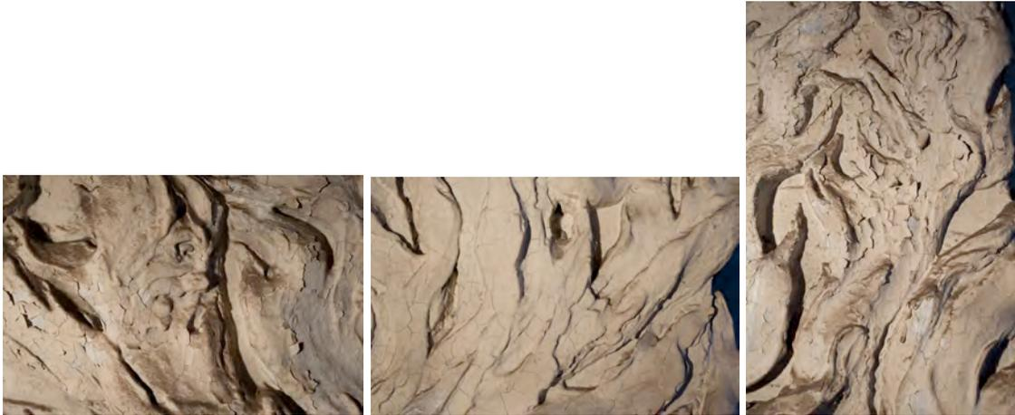
Figures 4a, 4b, 4c. Alligatoring, delimitation, and the resulting flaking and loss was visible through much of the white overpaint. Right: Level B, E Elevation; Center: Level A, E Elevation; Left: Level B, E Elevation. 2013.
